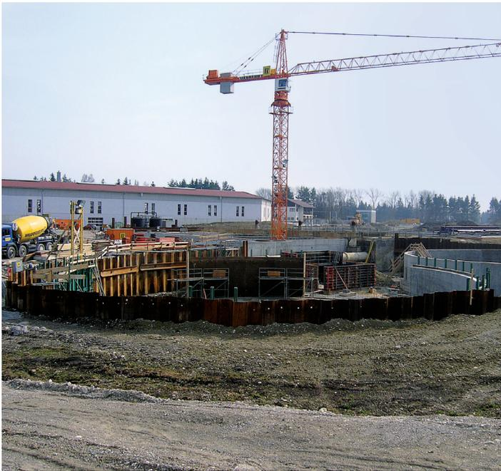
Treatment tank of a sewage treatment facility, made with CEM I 32,5 N-SR 3
