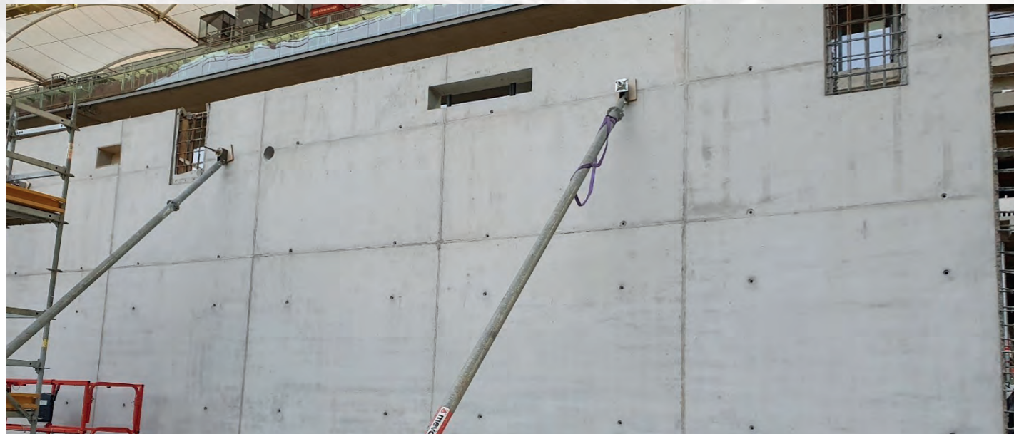
Picture: Concrete wall | construction site Mercedes-Benz Arena
