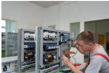
Toni Angermann, electrician | SCHWENK
