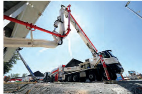
Concrete pump with secure support, BPD Vogtland | SCHWENK
