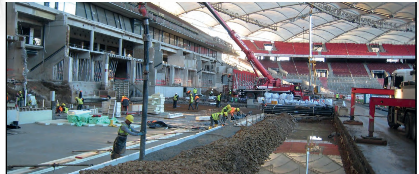
Picture: Construction site Mercedes-Benz Arena
