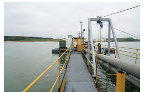
Dredger at the Borgsdorf plant | SCHWENK
