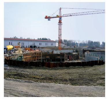
Treatment tank of a sewage treatment facility, made with CEM I 32,5 N-SR 3
